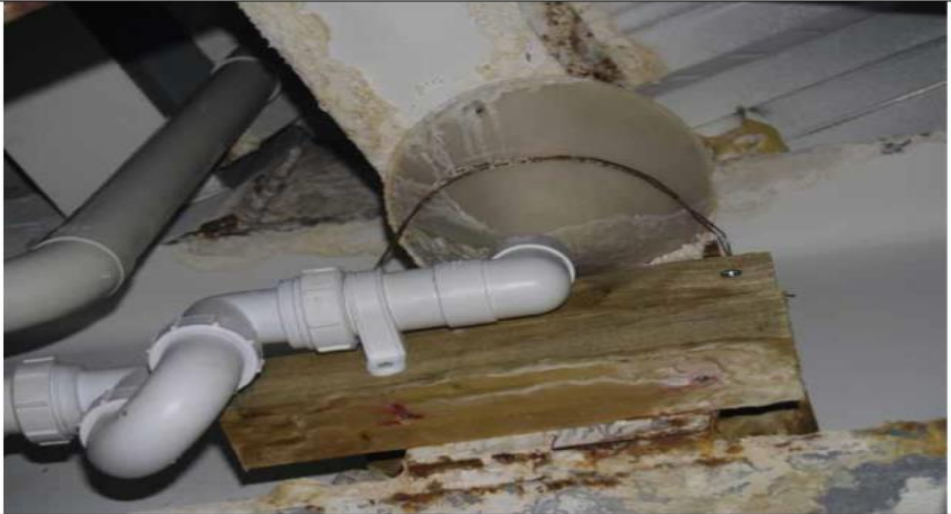
Domestic funnel wired in place by the contractor as catch vessel for major leak in ceiling void above changing area. Wire corroded and timber untreated
