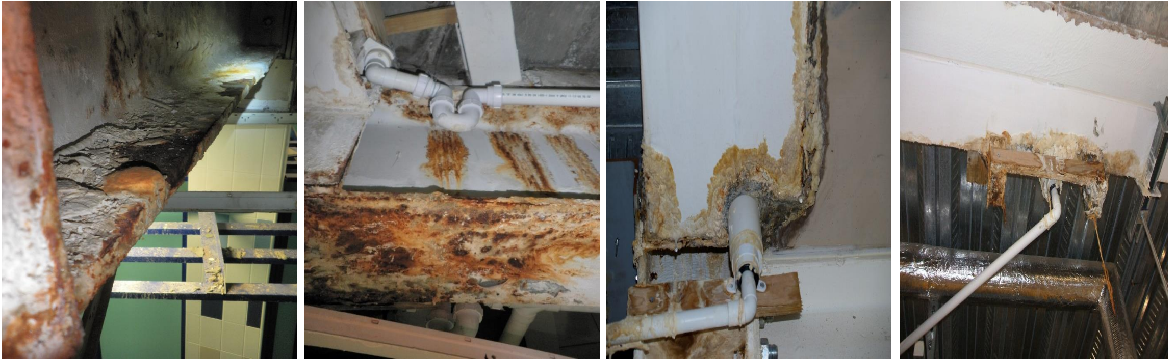
Impact of leaks from first floor area and corrosion to structural steelwork immediately below
