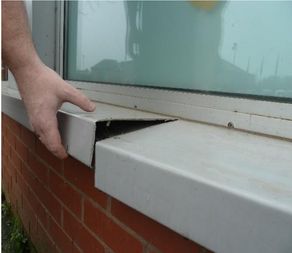
Poor external workmanship and detailing
