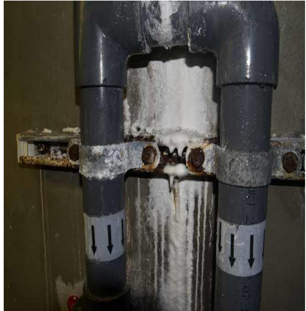
Examples of damage to pipe insulation and to galvanised fittings in plant room
