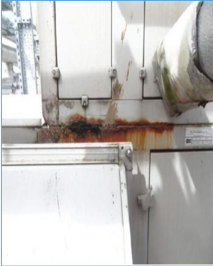
Examples of widespread corrosion to plant fittings including AHUs on roof
