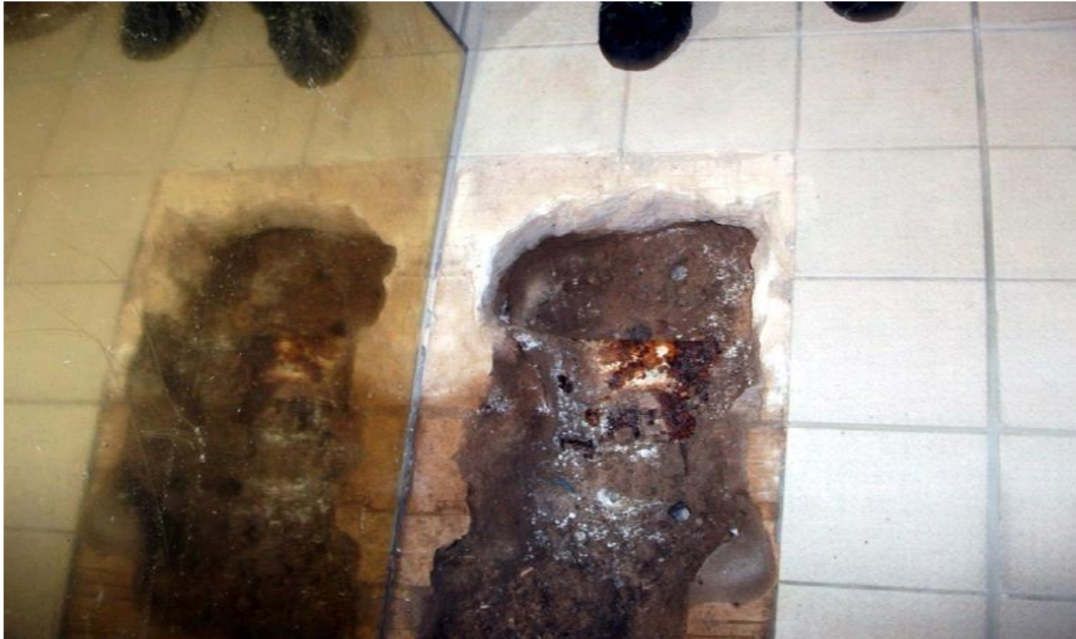
A corroded steel beam ( and its reflection in a mirror ) in the screed below an opened section of tiling.
