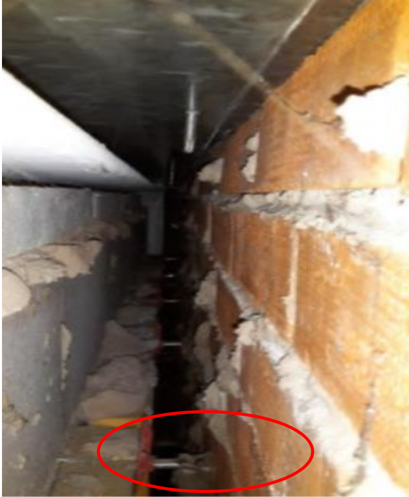
Wall ties not embedded in outer face and insulation missing
