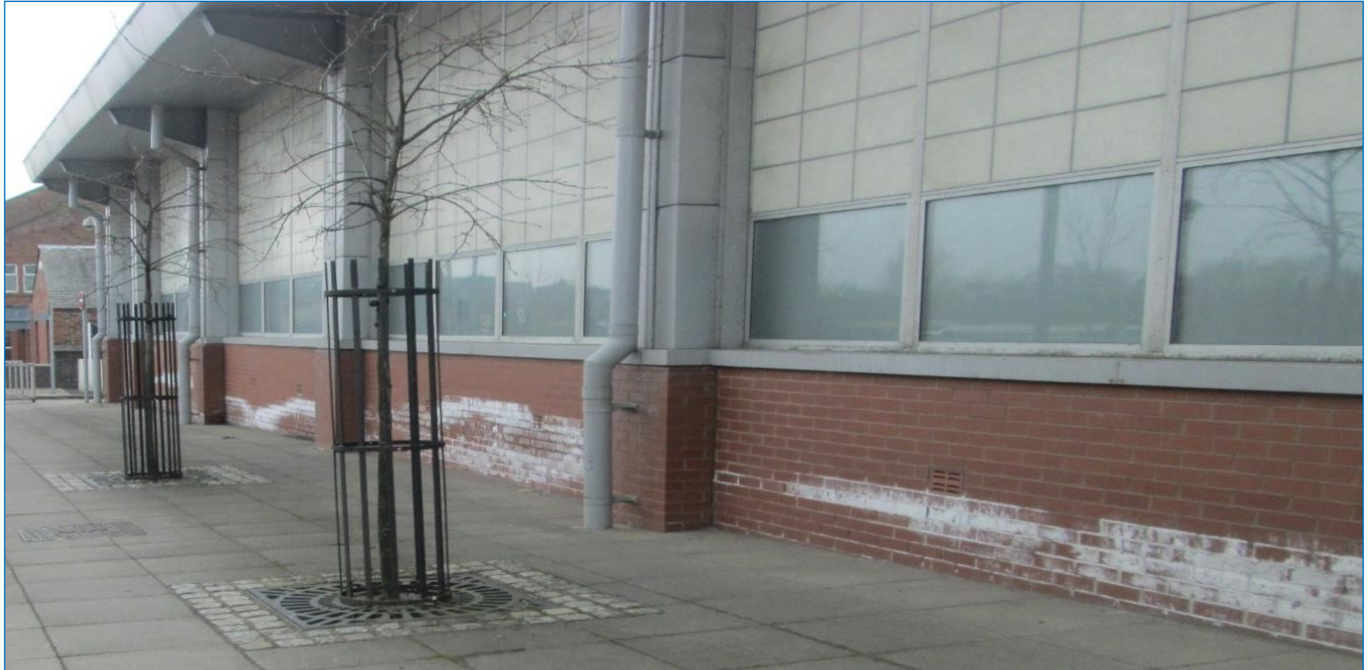
Street elevation of DG One building showing efflorescence due to constantly saturated wall
