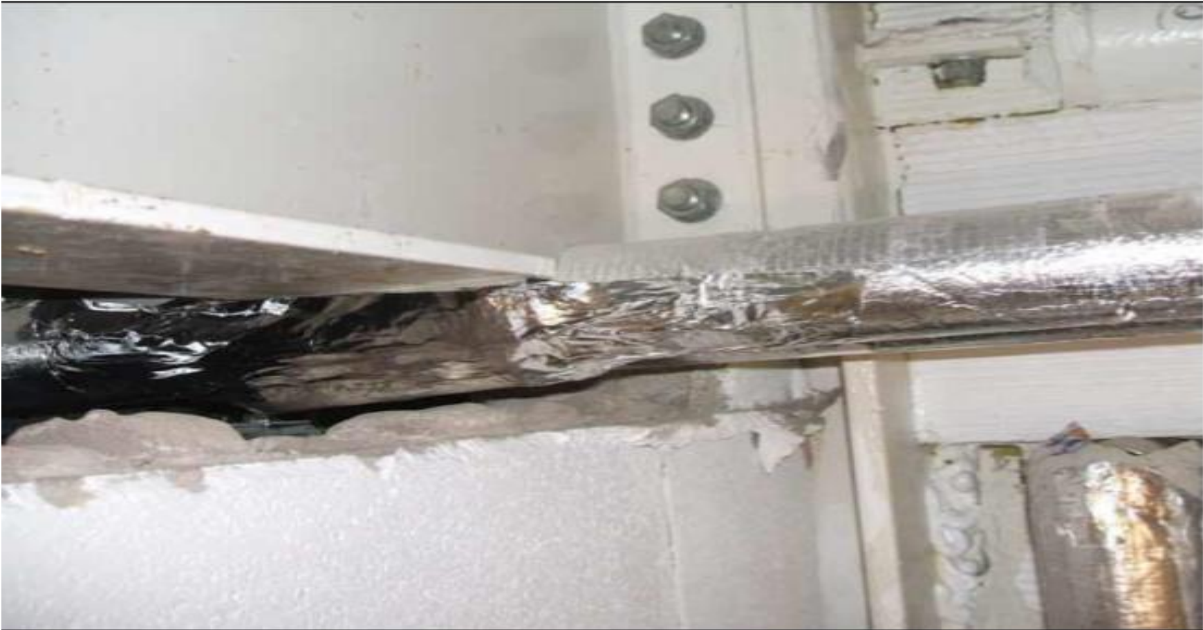
Unsealed hole as services pass through 1-hour fire resisting wall
