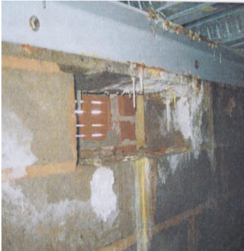
External and internal faces of saturated cavity wall
