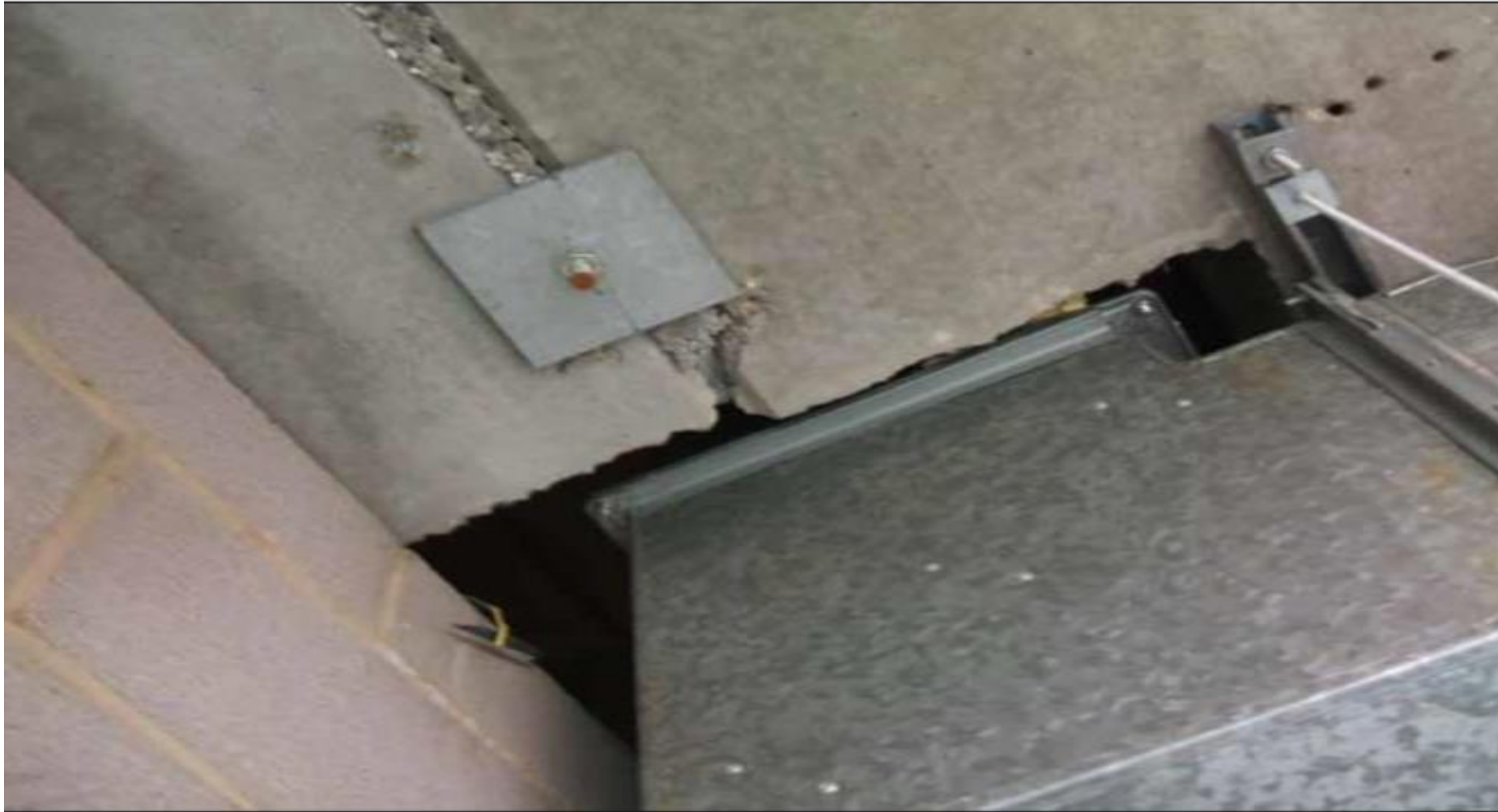
Ducts passing through plant room walls without fire or smoke seals
