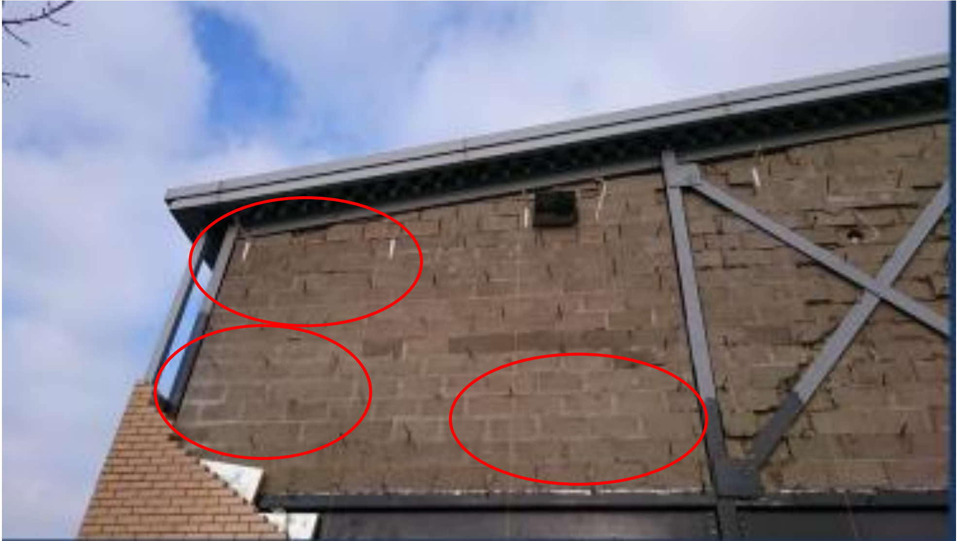
Areas of wall-tie spacing not as it should be with ties pulled out or not there in first place
