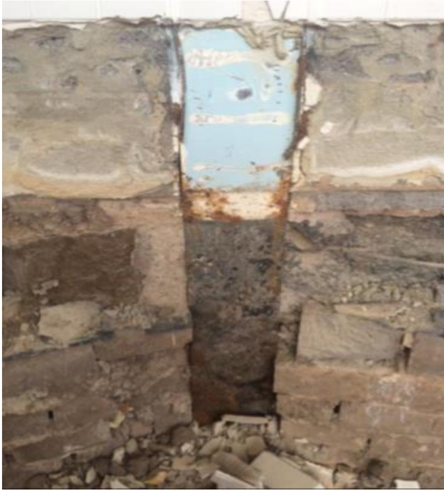
Corroded underfloor sections of steel columns
