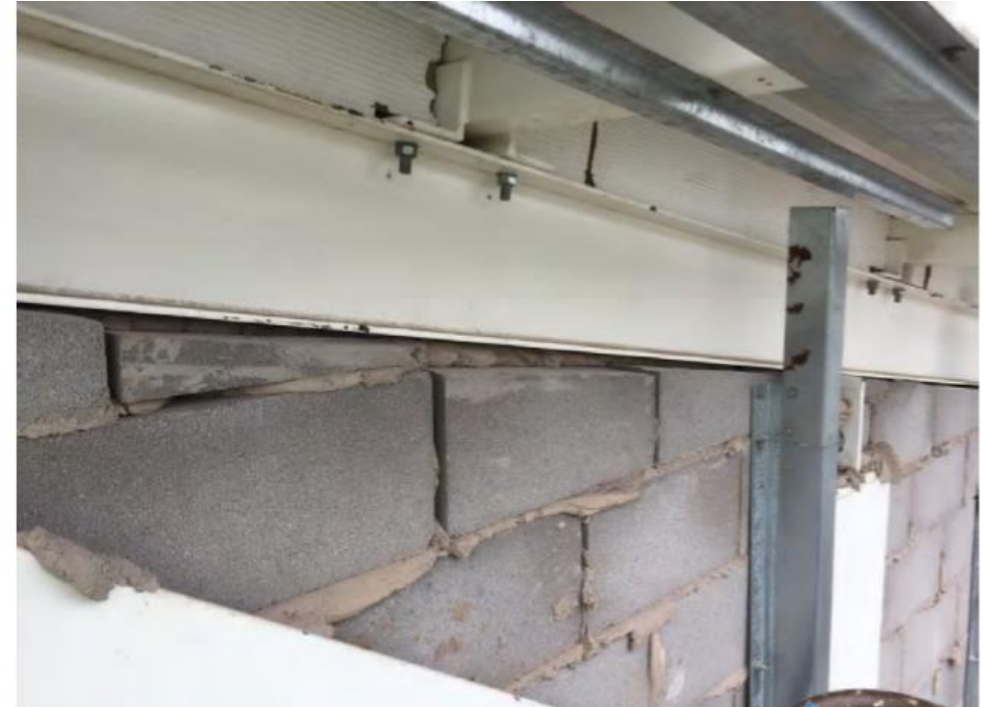
No supports to head of blockwork and inadequate supports for external cladding
