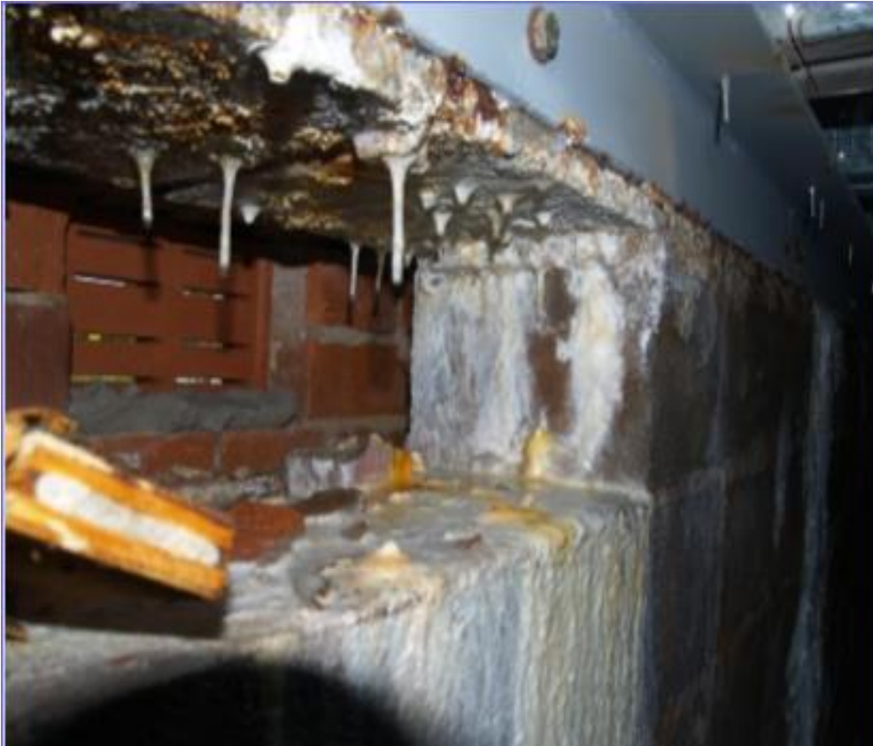
Saturated damp and efflorescence in void under pool area
