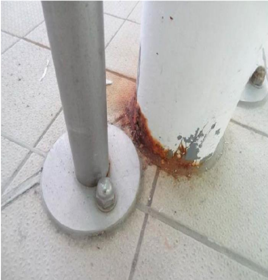
Corrosion of metal fittings throughout building
