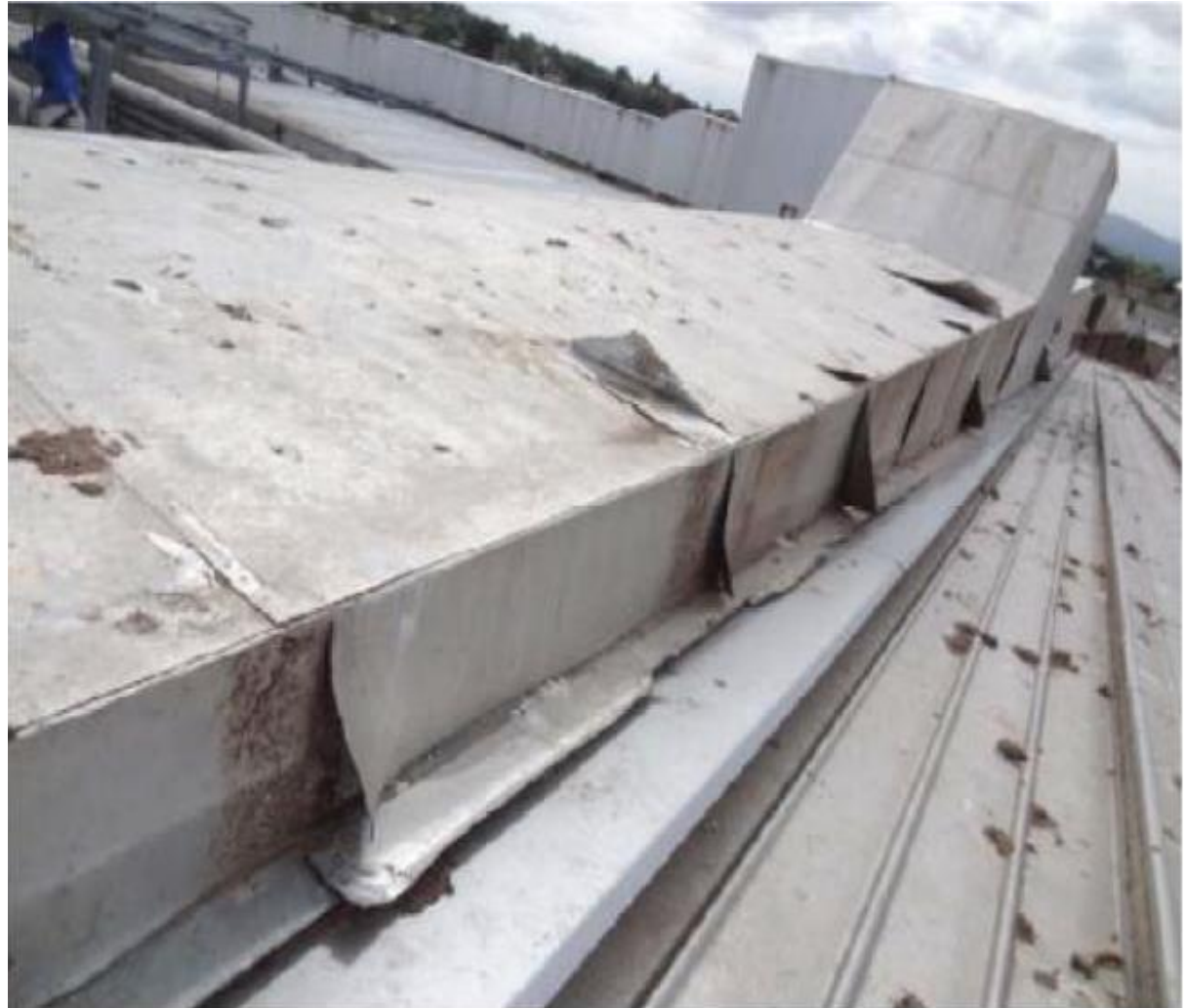
Potentially dangerous delaminating coverings to roof ducts
