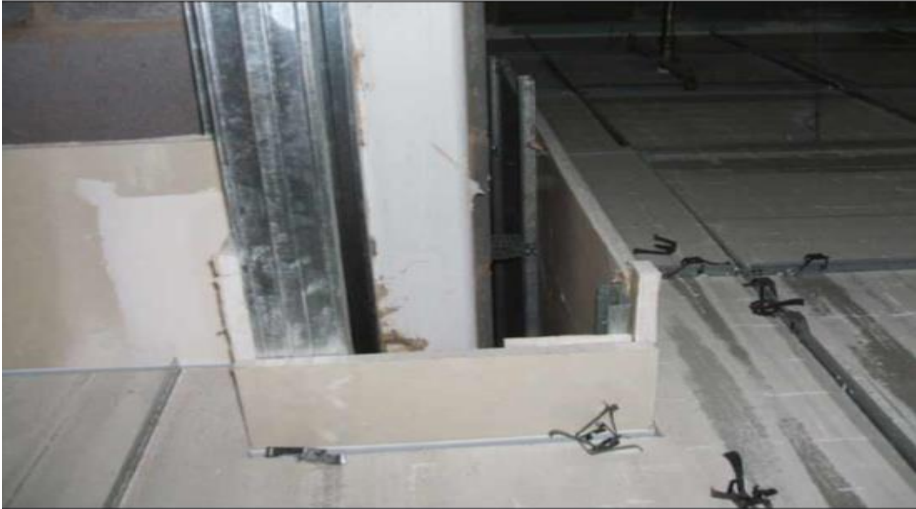
Void to lift shaft and floor below not fire or smoke sealed
