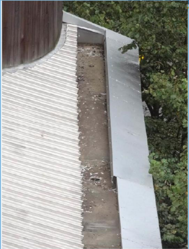
Poorly fitted and sealed flashing
