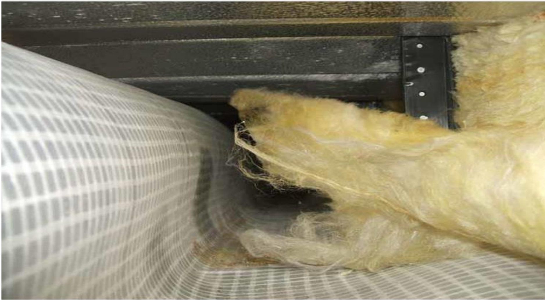
Continuous gap of insulation at eaves
