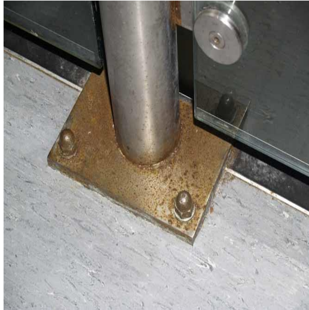
Examples of corrosion to steel fittings throughout the wet area found to be 304 grade steel as opposed to specified grade 316
