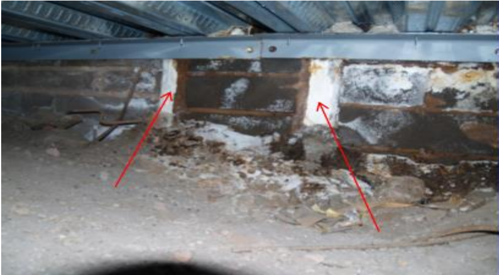
Steel columns indicated with red arrows are rusted and corroded
