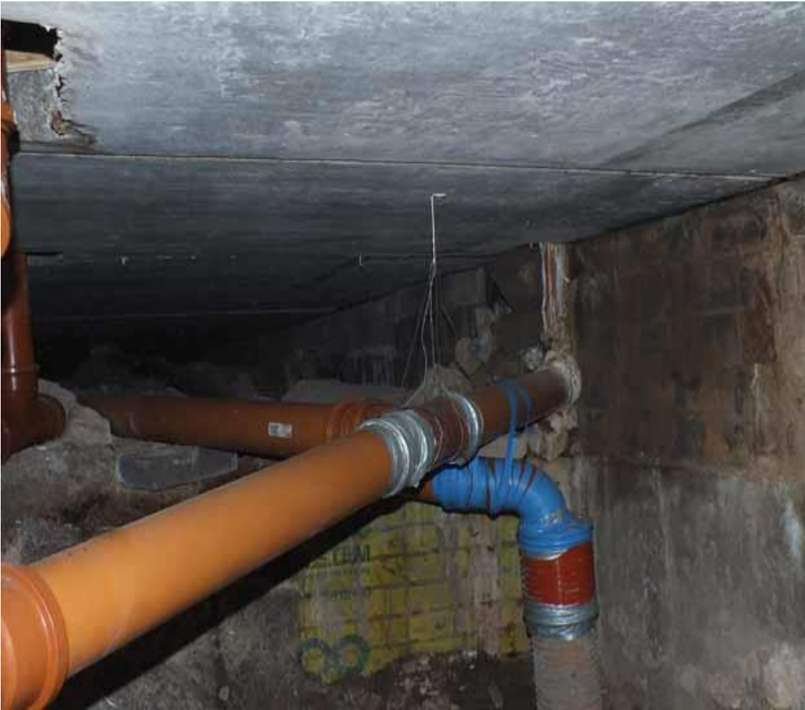
Examples of inadequately joined, supported and sealed drainage in the building voids under DG One
