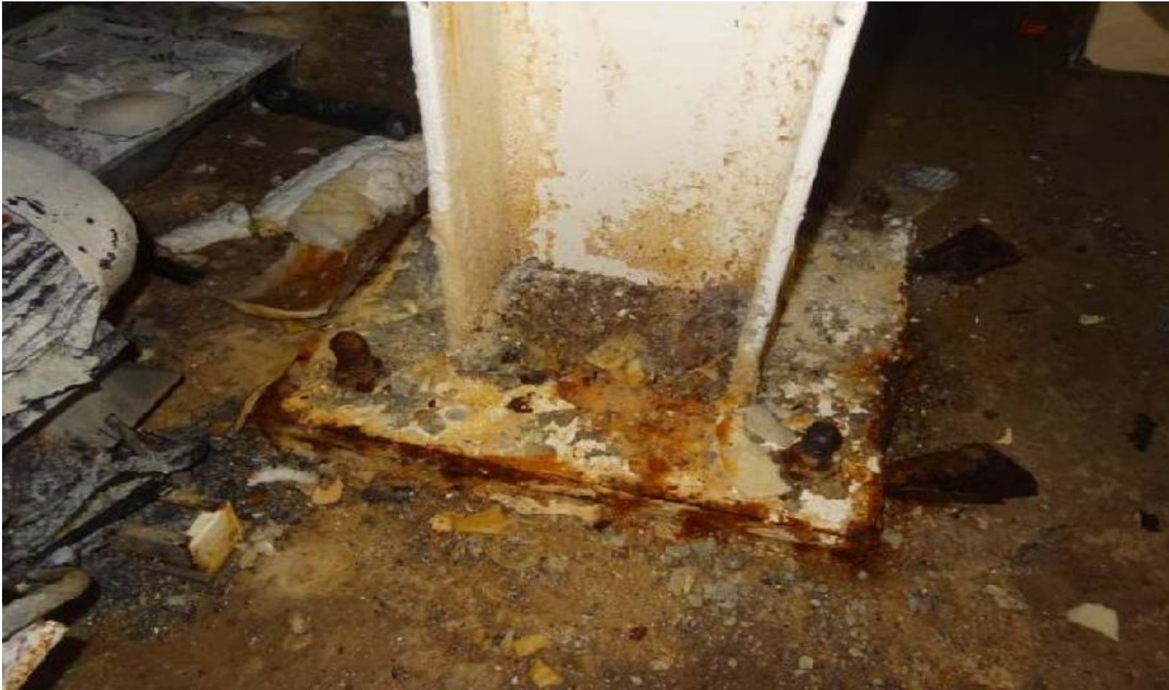
Corroded base of steel column in main plantroom
