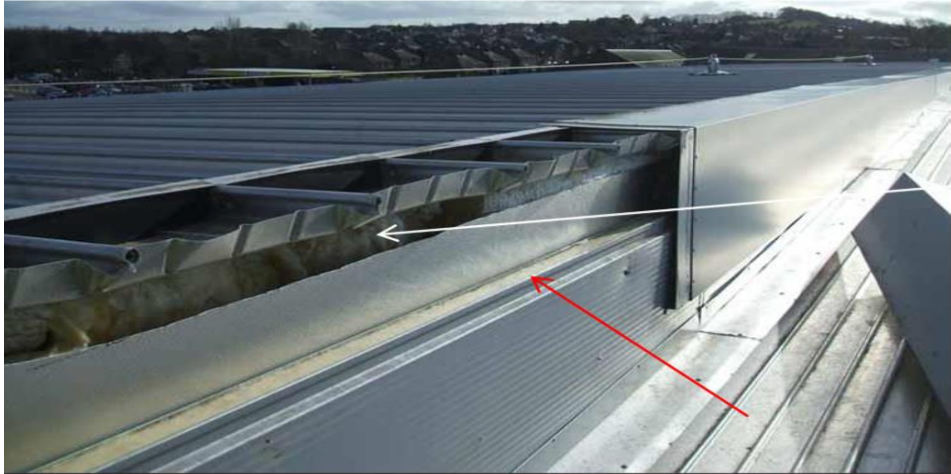
Large gap between roof and wall insulation
