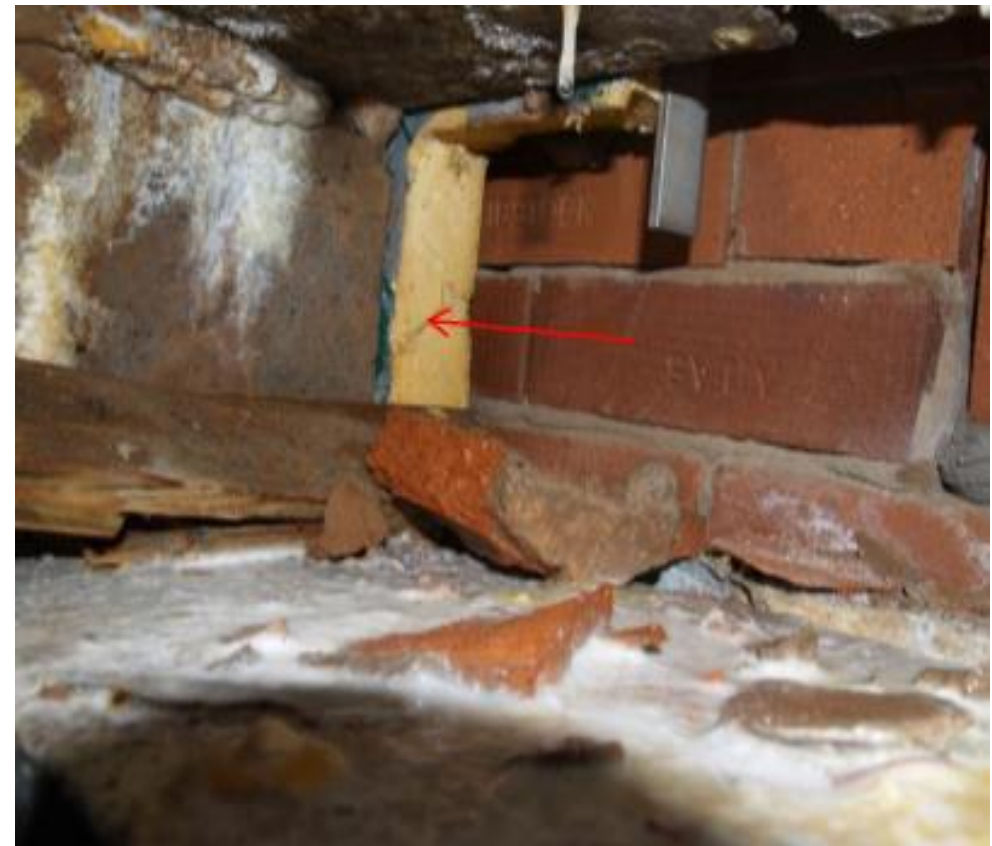
Saturated damp and efflorescence in void under pool area
