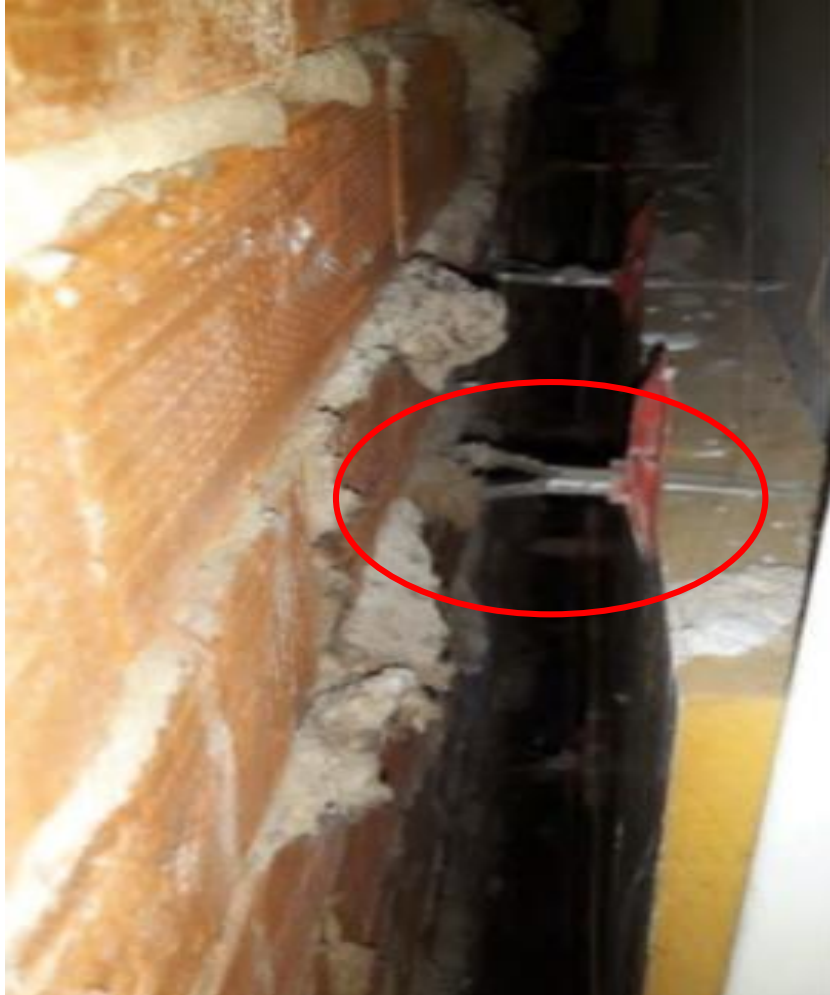
Wall ties not embedded in outer face and insulation missing
