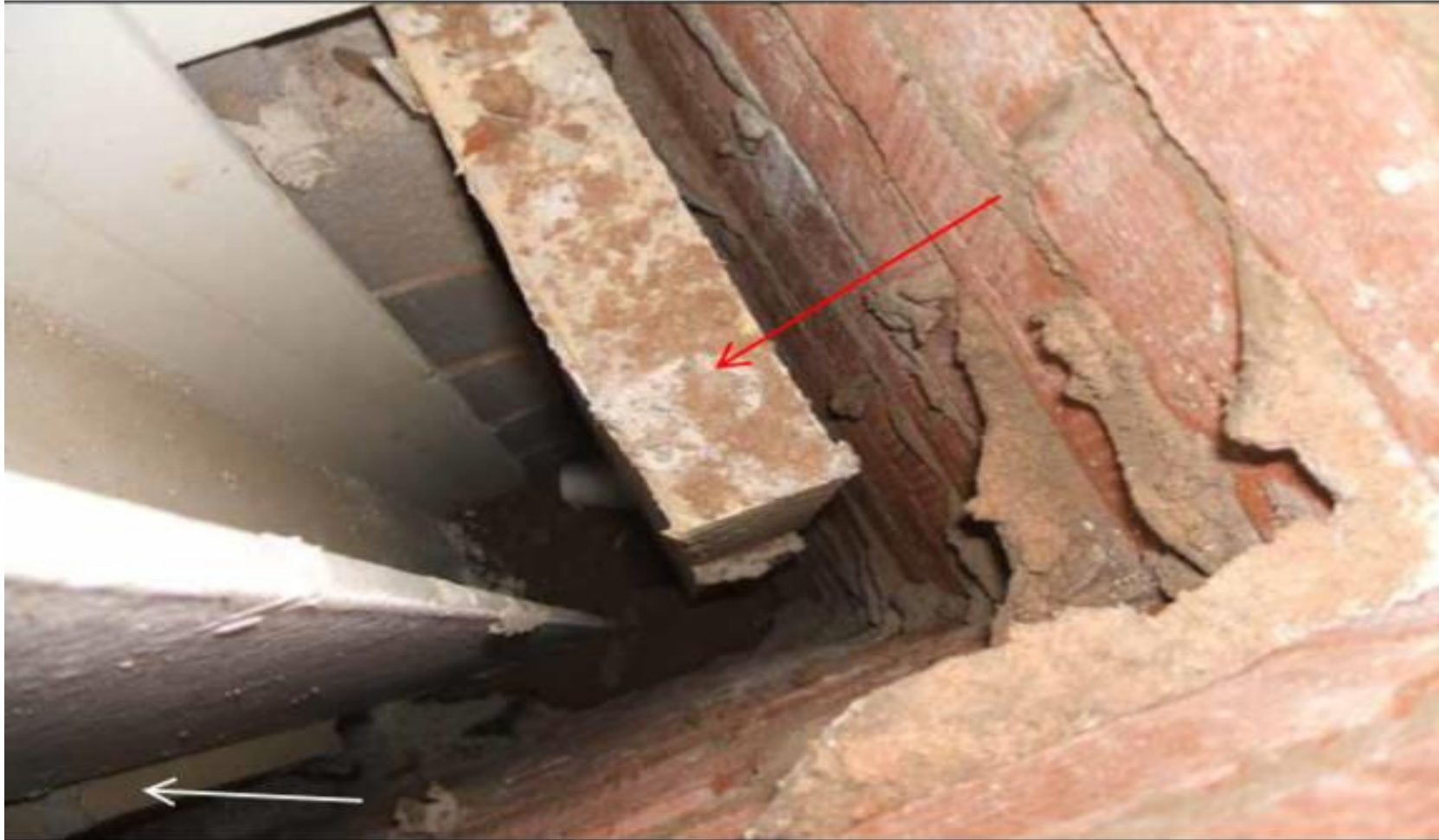
Isolated pieces of insulation below floor level but none above and through corner where cold bridge occurs at steel column
