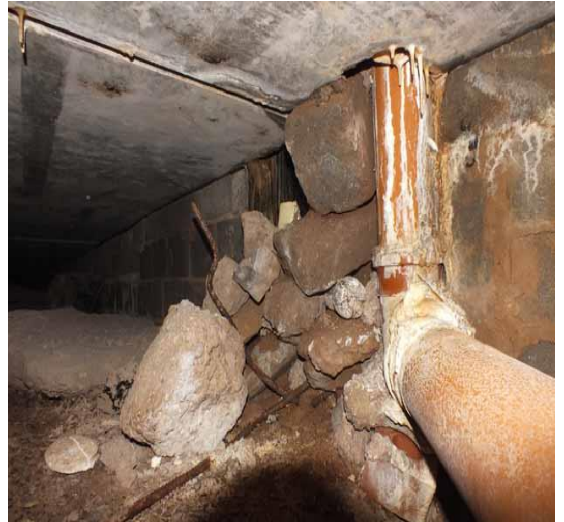
Examples of inadequately joined, supported and sealed drainage in the building voids under DG One
