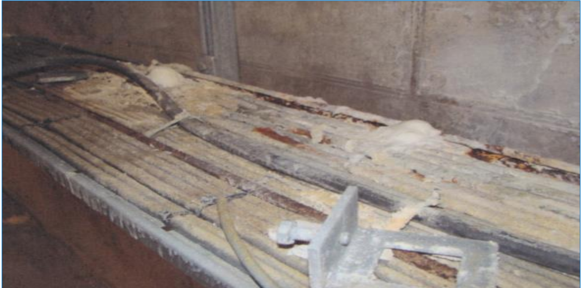
Severe corrosion evident to electrical and mechanical services from leaking pool chemicals and condensation
