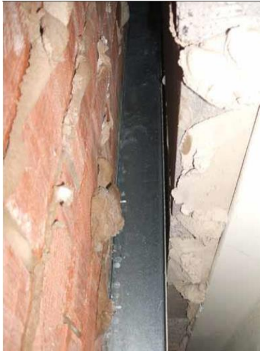
External wall Insulation missing
