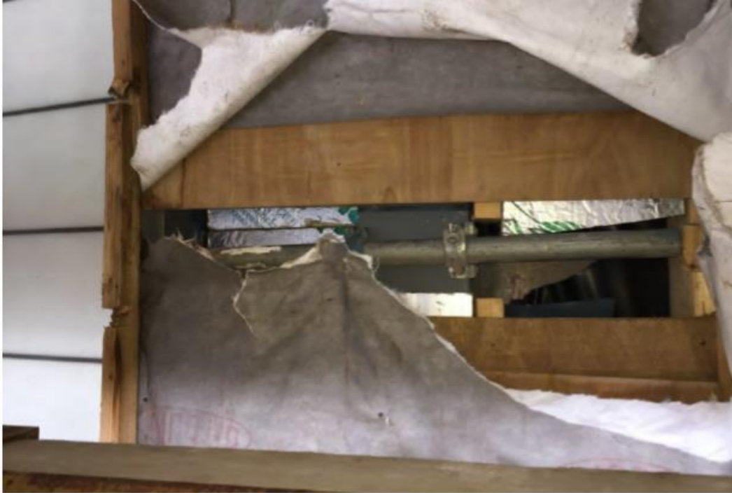
Scaffold tube remaining from original construction revealed on removal of cladding. Timber and insulation boded around tube
