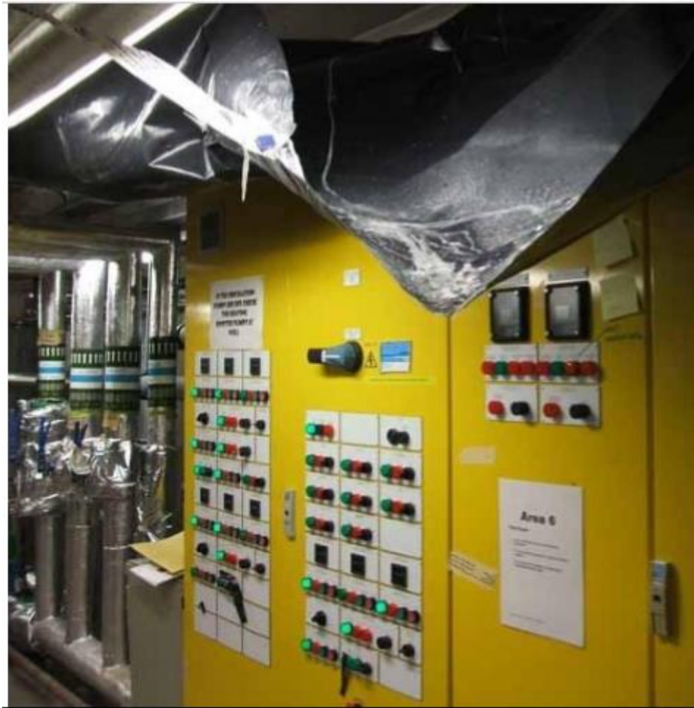
Polythene sheeting protecting electrical switchgear from overhead water leakage caught in carefully positioned bucket
