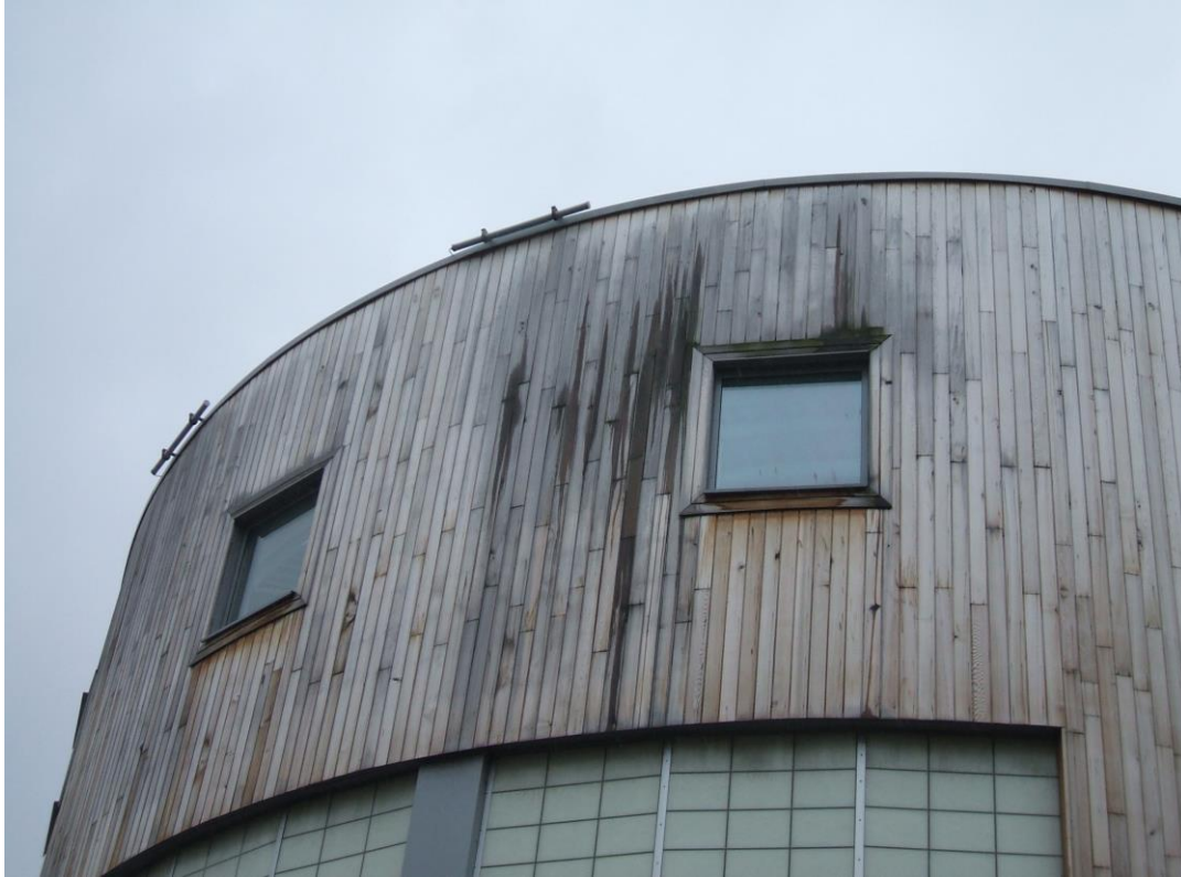
Uneven staining of timber cladding
