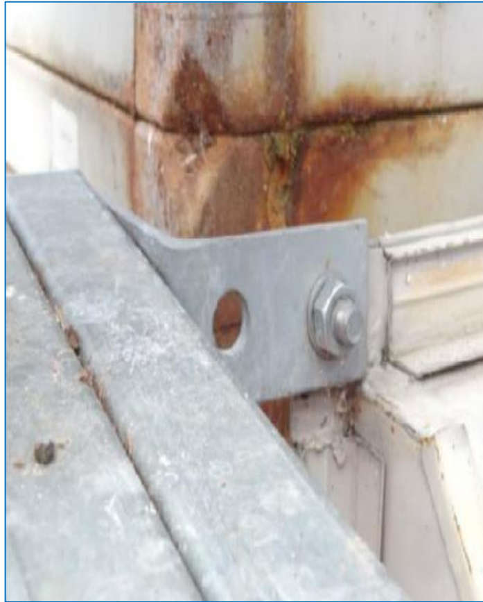
Examples of widespread corrosion to plant fittings including AHUs on roof
