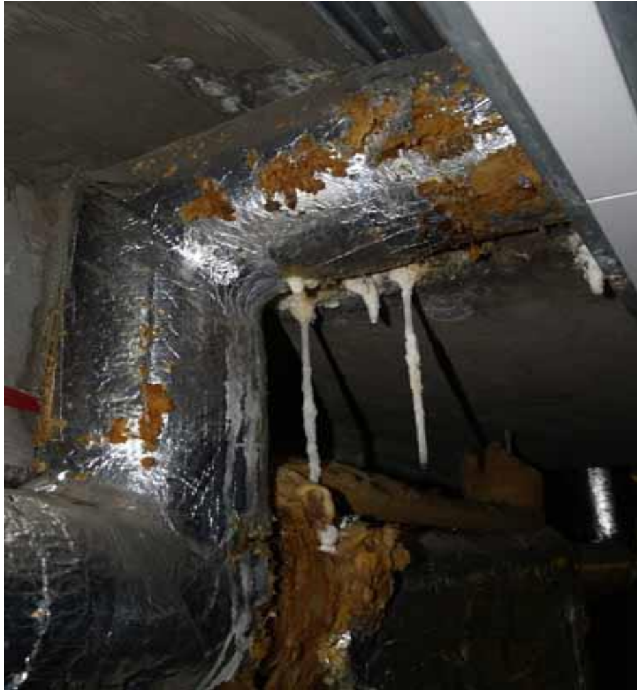
Examples of damage to pipe insulation and to galvanised fittings in plant room
