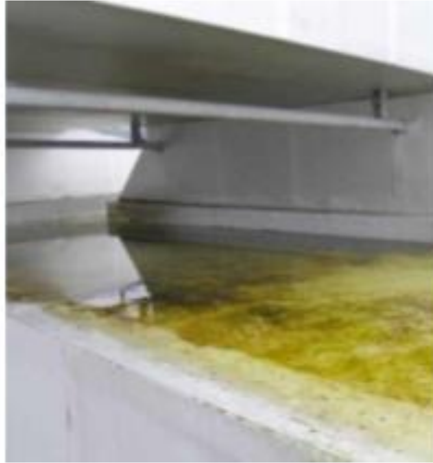
Discharge from dance studio roof directly onto pvc membrane and ponding due to ineffective drainage
