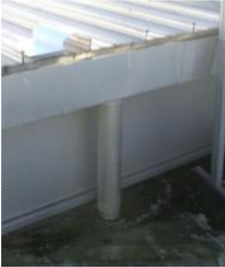
Discharge from dance studio roof directly onto pvc membrane and ponding due to ineffective drainage
